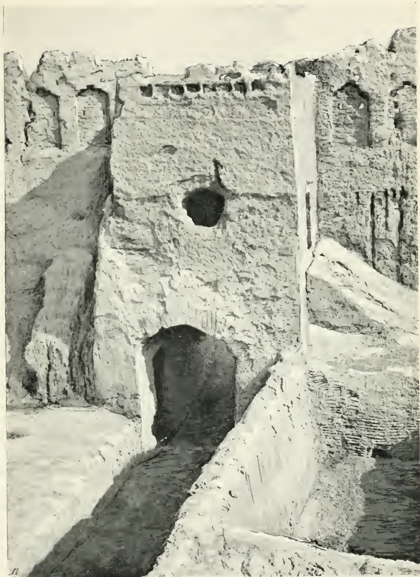
THE GATE OF RUSTAM'S CITY, as seen from Rustam's House.
